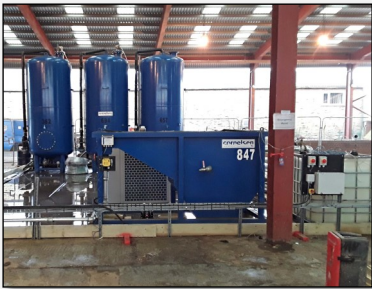
Water Treatment Plant
