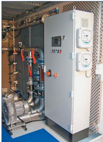
ATEX Rated SVE system with Automated Dilution Air & Soil Gas valves for optimised CatOx treatment
