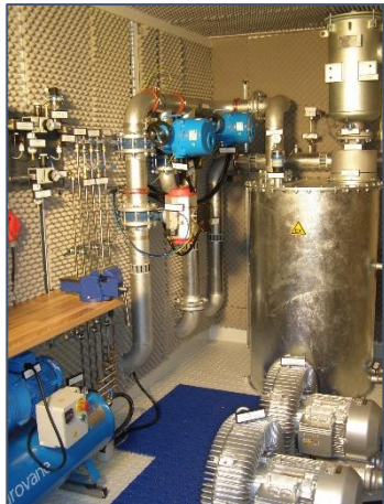
ATEX Rated SVE system with Automated Dilution Air & Soil Gas valves for optimised CatOx treatment
